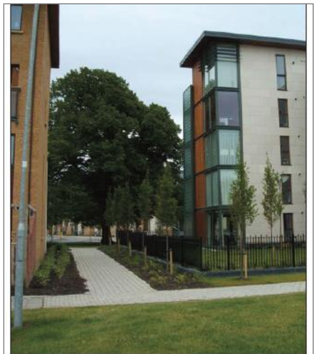
Figure 3.23: Examples of vehicular cul-de-sacs in Adamstown, Co. Dublin, which allows for through pedestrian and cyclist access only and has incorporated design measures to ensure that it is safe (i.e. clear sightlines and passive surveillance).
